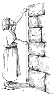
LB00125 Builder using plumbline
